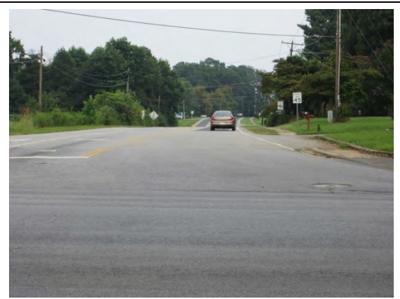
Looking east towards Lee Avenue from the US 601 intersection
