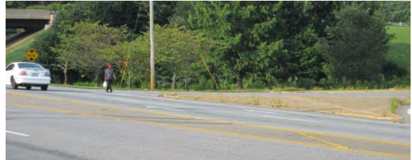
Photo showing pedestrian coming from underpass and crossing SB US 421 entrance ramp.
