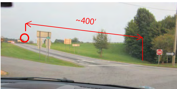
Photo illustrates distance from US 421 NB Off-Ramp terminus at US 601 to existing WRONG WAY (R5-1a) signs.
