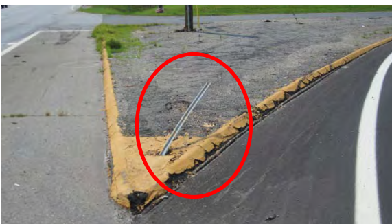
Photo showing bent sign post and missing sign at raised channelizing island at US 421 NB On Ramp.
