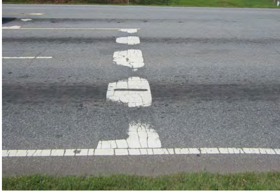
Photo showing worn pavement markings along US 601 near the NB US 421 ramps.
