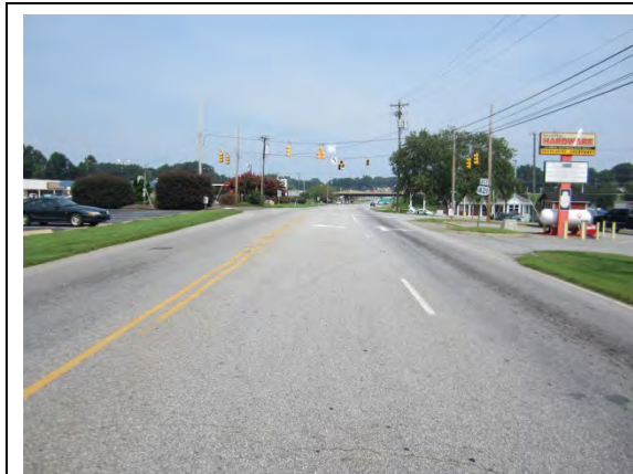
Looking north along US 601 towards the Sharon Road intersection
