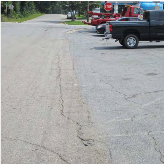
Photo showing uninhibited access for the Shell station along Maple Street.
