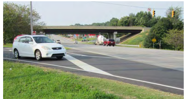
Photo showing right-turning driver looking over her shoulder in light of the sharp angle between the US 421 SB Off-Ramp right-turn movement and US 601.
