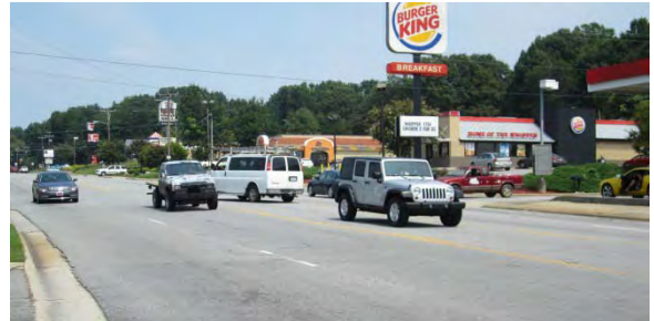
Photo showing conflicting northbound and southbound left turns from the US 601 two-way left-turn lane just south of Beroth Drive.
