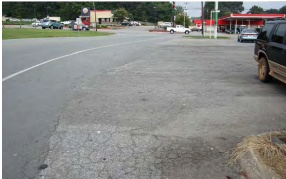
Photo showing uninhibited access for the BP station along Beroth Drive.
