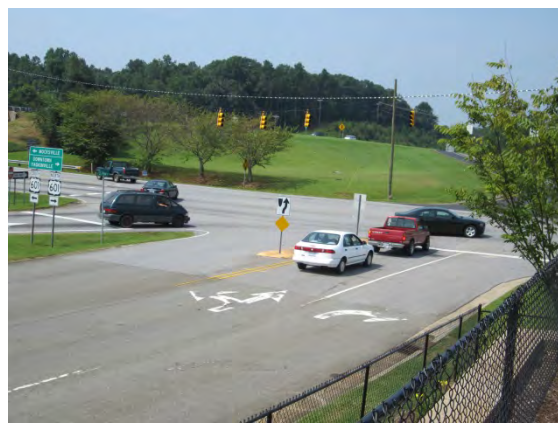
Looking west along Pine Street at the US 601 intersection
