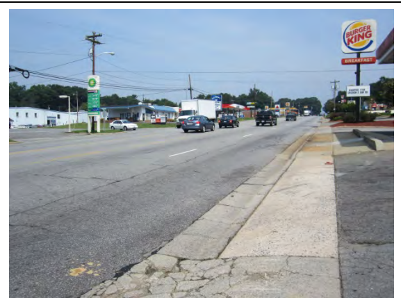
Looking north along US 601 towards the Beroth Drive intersection
